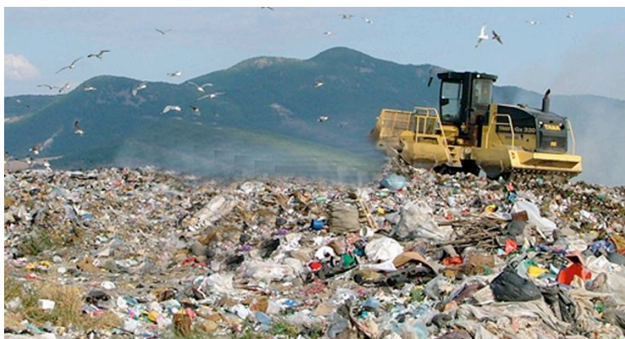
Figure 4. Aleko Konstantinovo open dump rehabilitation studies
