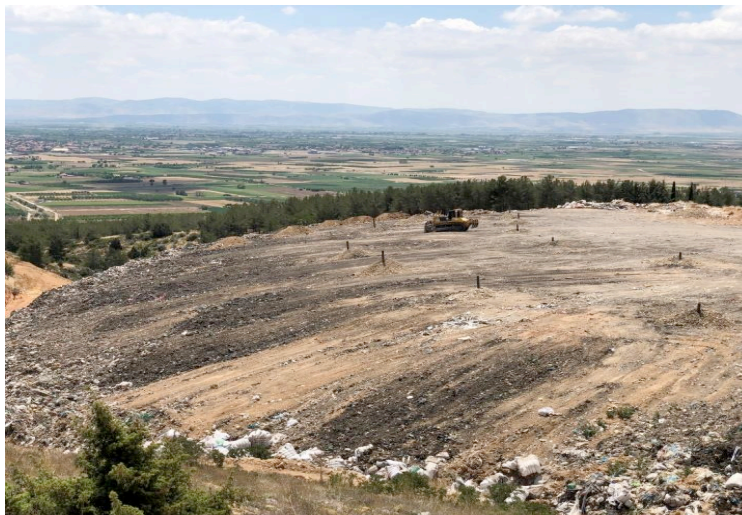
Figure 1. Installation of gas chimney
